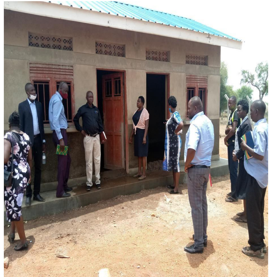
Joint monitoring at power house during construction
