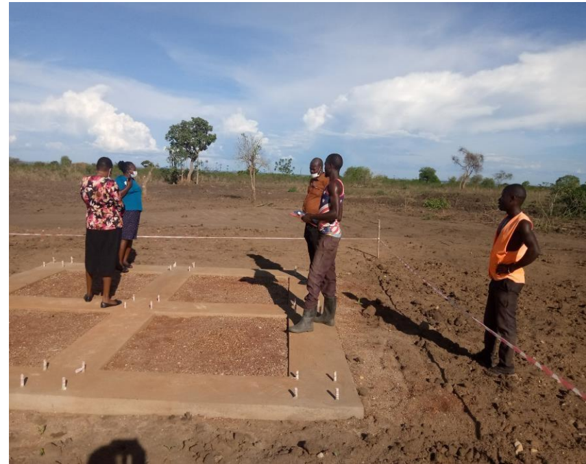
Joint technical supervision of reservoir foundation
