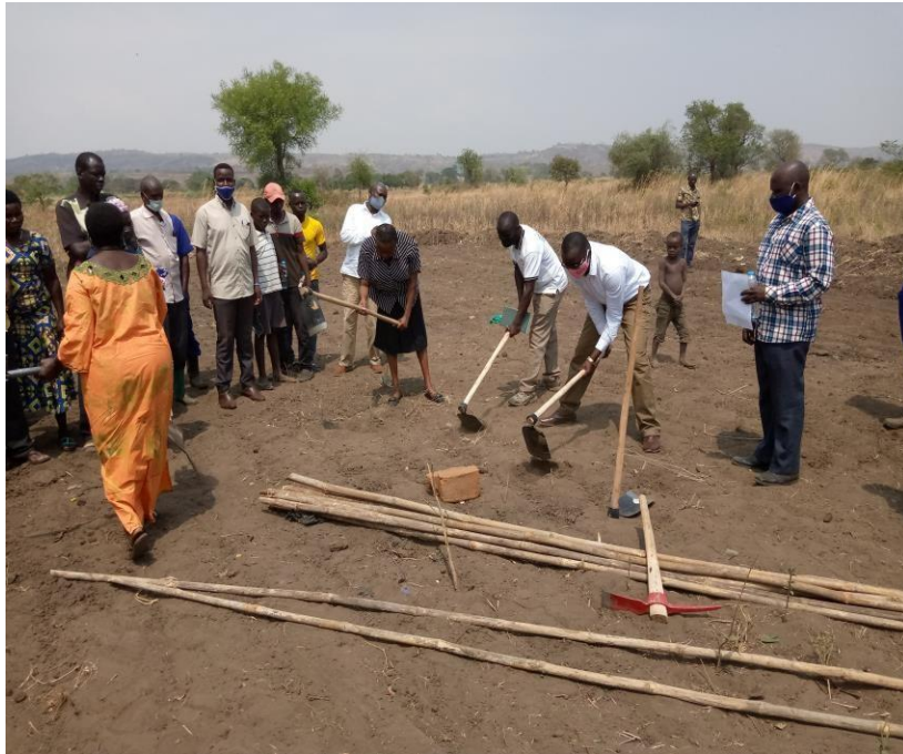
Project ground breaking with political leaders
