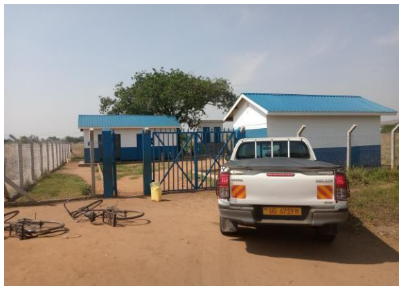
Completed power house & pump attendant house
