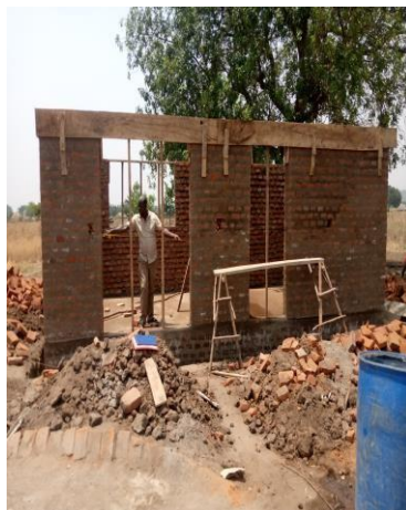
Power house at construction
