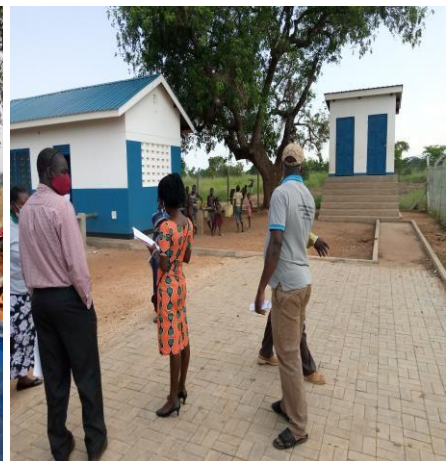
Completed power house and ecosan toilet
