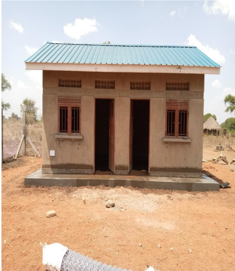
The guard/pump attendant house under construction
