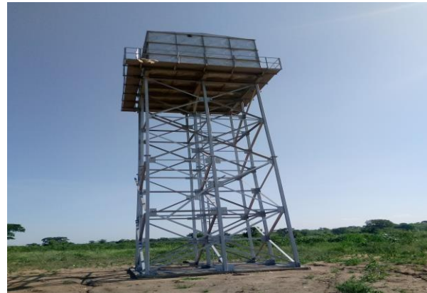
The completed reservoir
